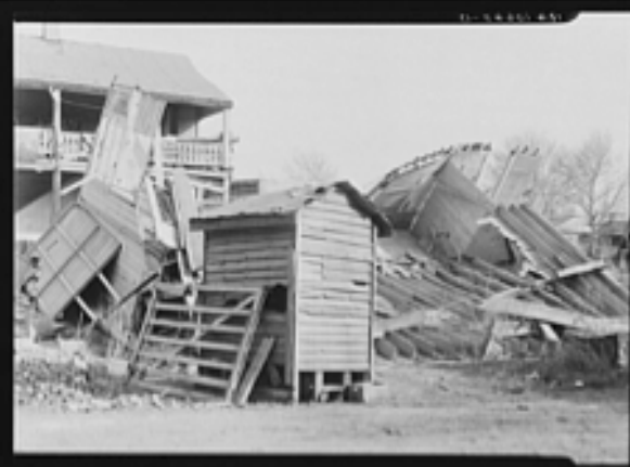
Flood damage. Shawneetown, Illinois
